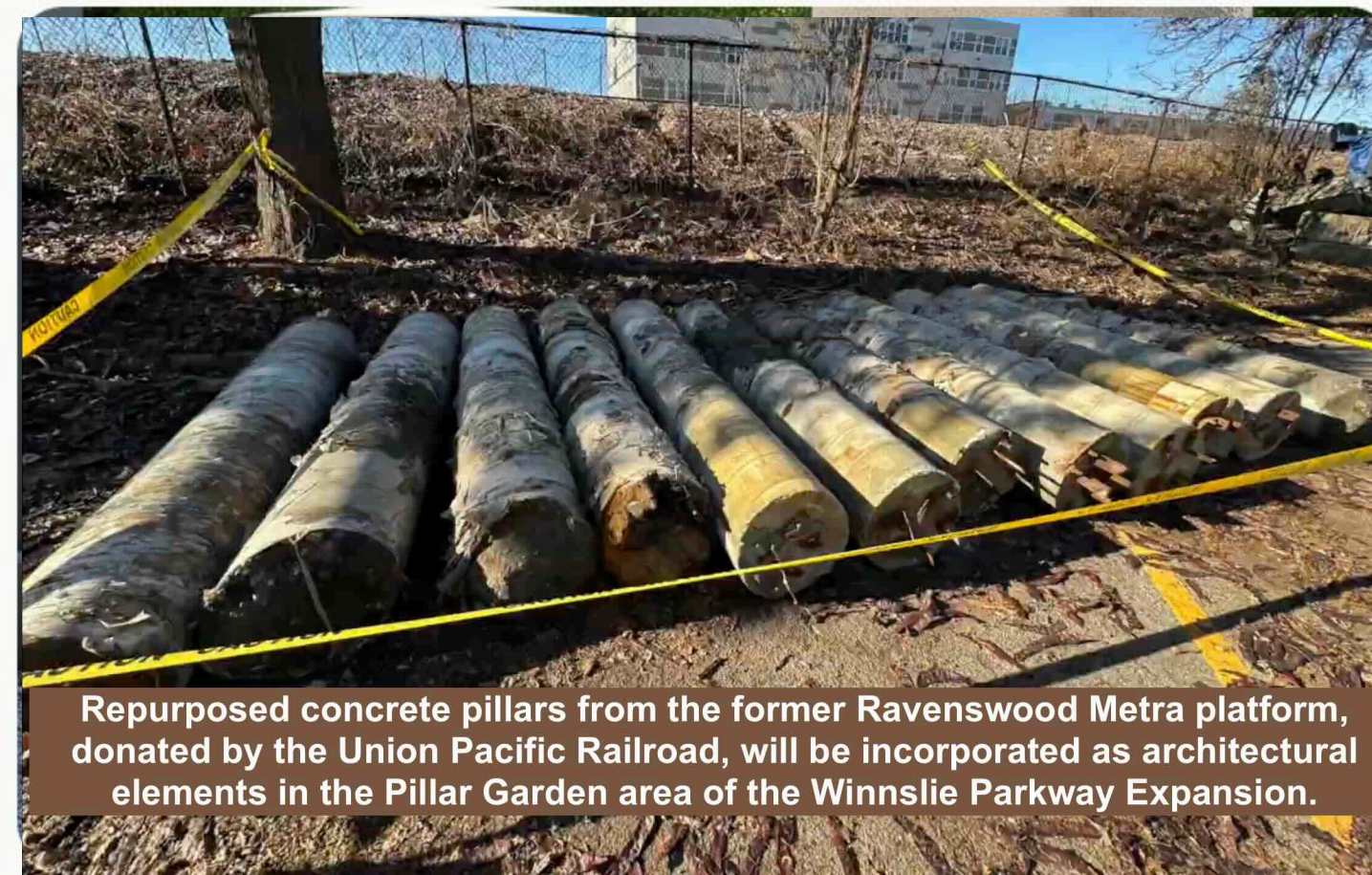
Repurposed Materials: Concrete pillars from the former Metra platform, donated by Union Pacific, serve as architectural elements.
